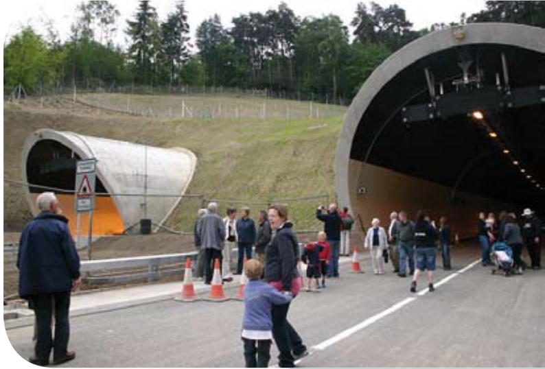
The Hindhead Tunnel which is due for completion in July 2011
